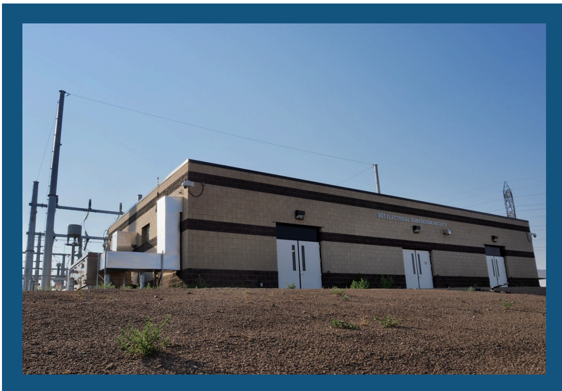
Support building for the new electrical substation at Metro Water Recovery's RWHTF in Denver, CO
