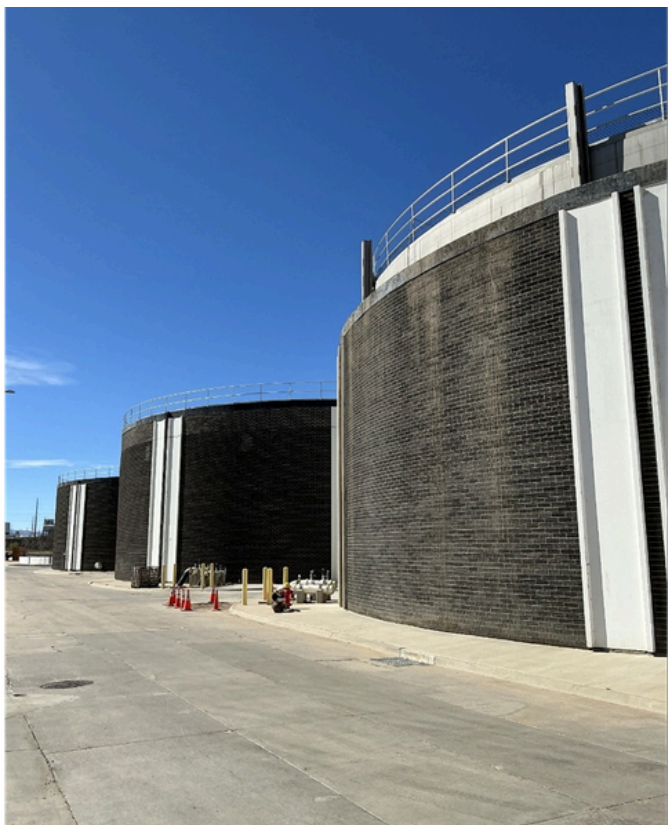
Figure 3 – Anaerobic digesters at RWHTF
