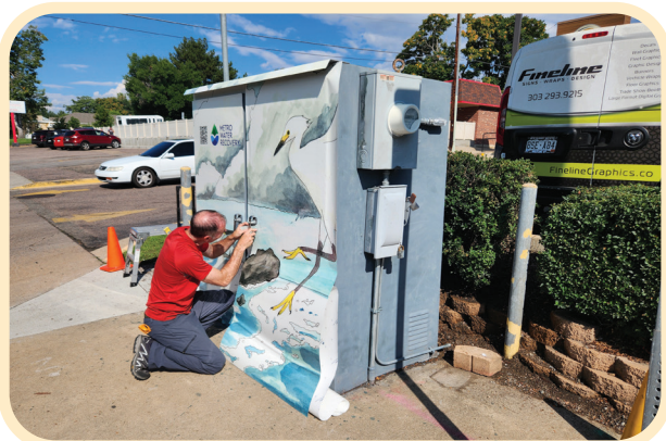
A contractor applies the vinyl wrap to the utility cabinet.
