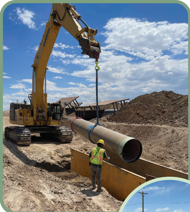
A pipe is lowered into place during construction.
