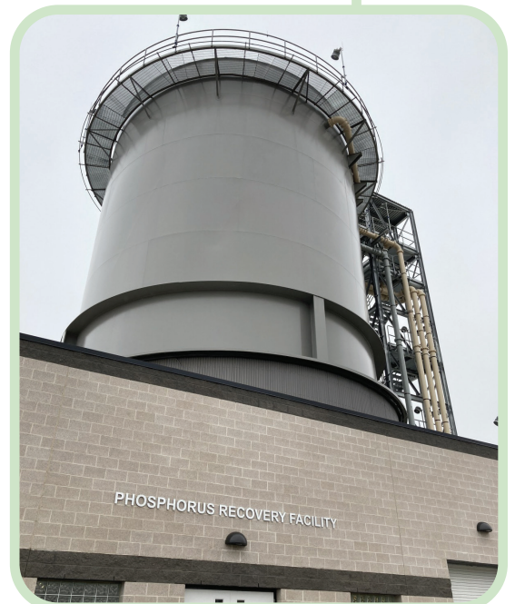
Metro's MagPrex™ phosphorous recovery reactor at RWHTF.
