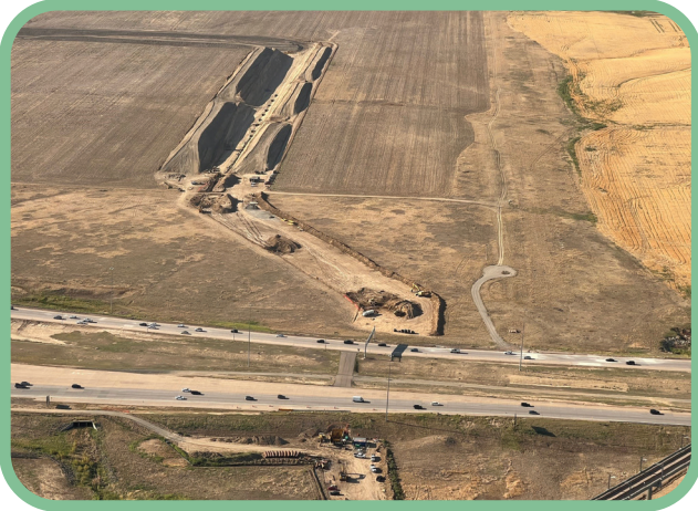
Second Creek pipeline construction.
