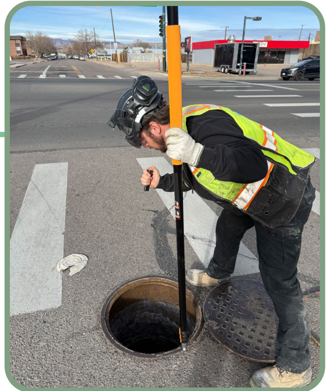
In the field inspecting Metro's sewer lines
