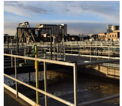
Aeration basins at the Robert W. Hite Treatment facility in Denver.
