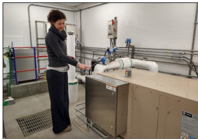
Chief Innovation Officer Tanja Rauch-Williams points to the heat pump in the OSCB Heat Recovery Shed, with the heat exchanger behind her, to the right of the broom.
