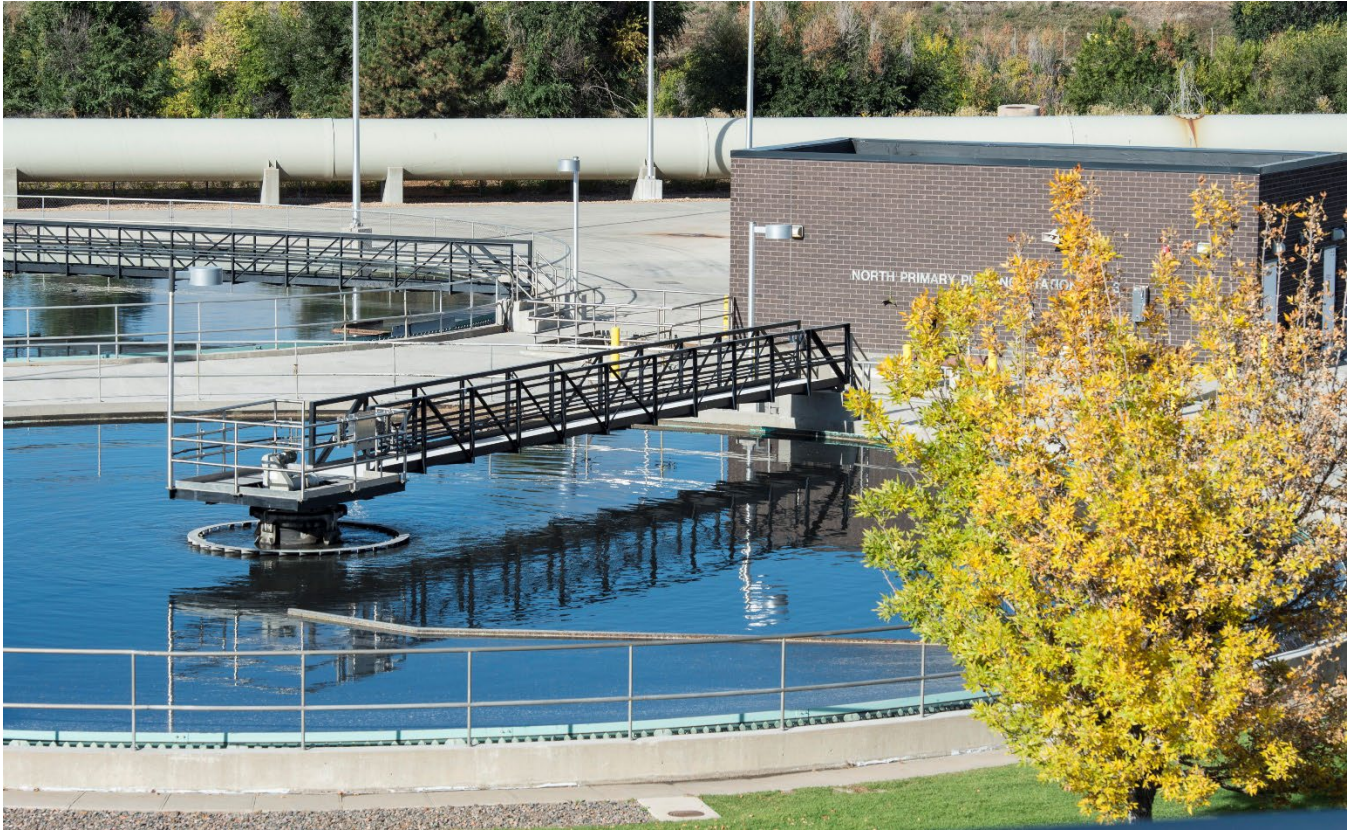
Robert W. Hite Treatment Facility in Autumn.
