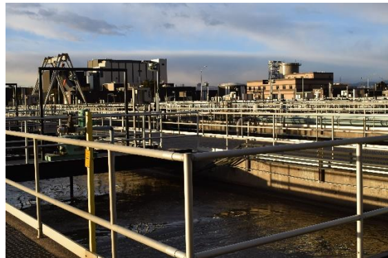
The aeration basis at the Robert W. Hite Treatment Facility in Denver
