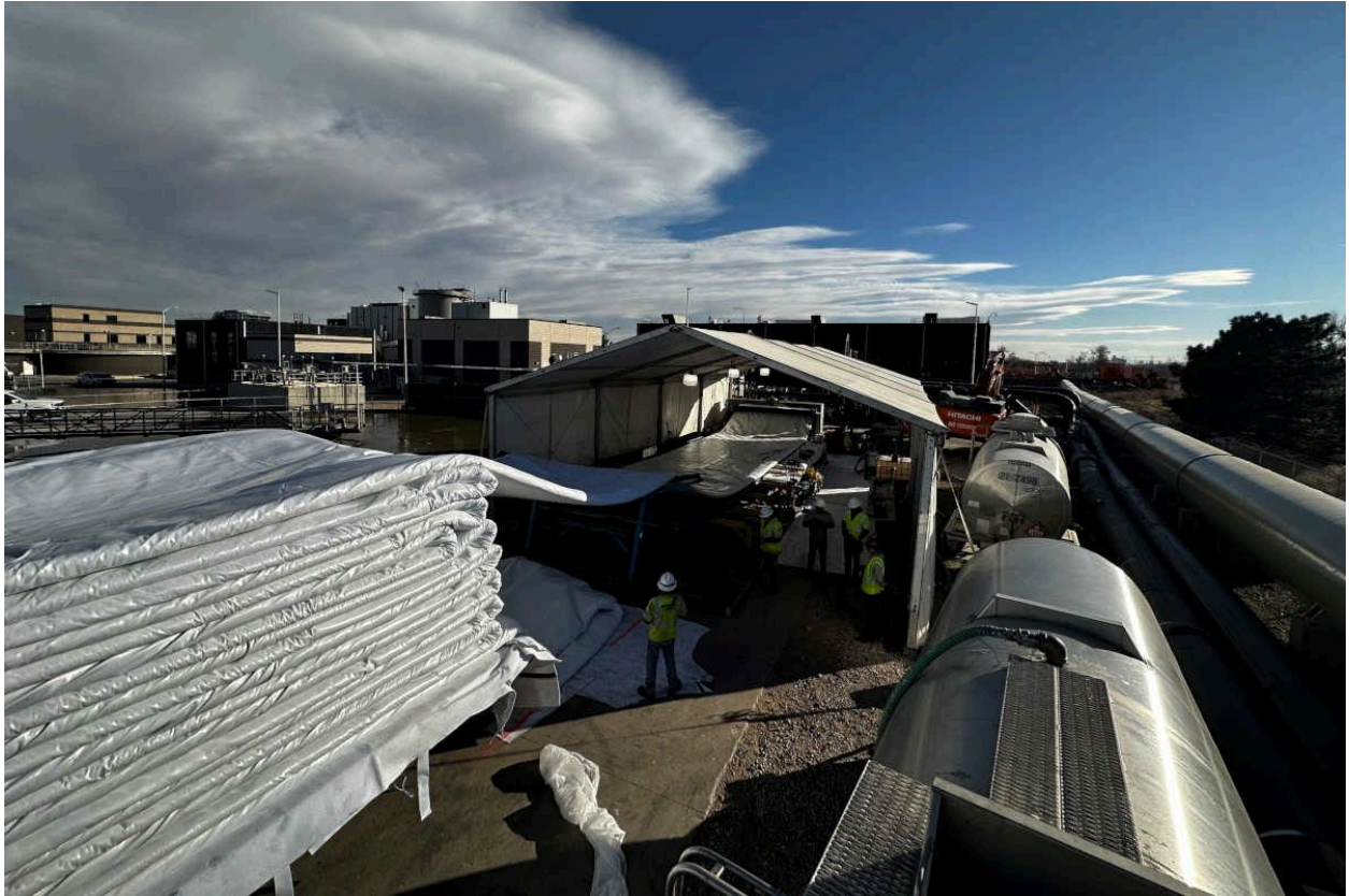
Robert W. Hite Treatment Facility in 2023. Trenchless technology.
