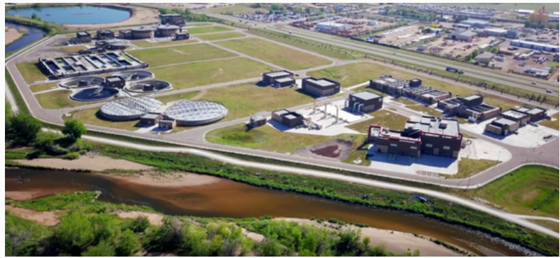
Top: Headworks area at Metro's Robert W. Hite Treatment Facility, where Metro treats and reclaims about 130 million gallons of wastewater per day. Below: Aerial view of Metro's Northern Treatment Plant in Brighton.
