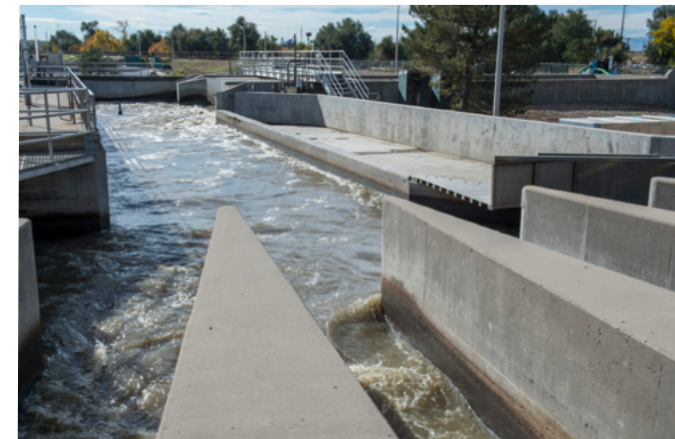
RWHTF influent channels.
