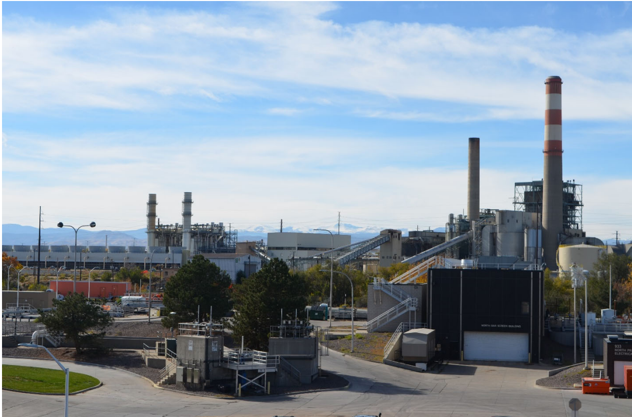
Robert W Hite Treatment Plant, taken in 2022
