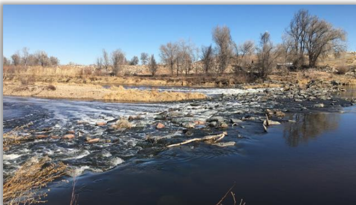
Repaired grade control structure
