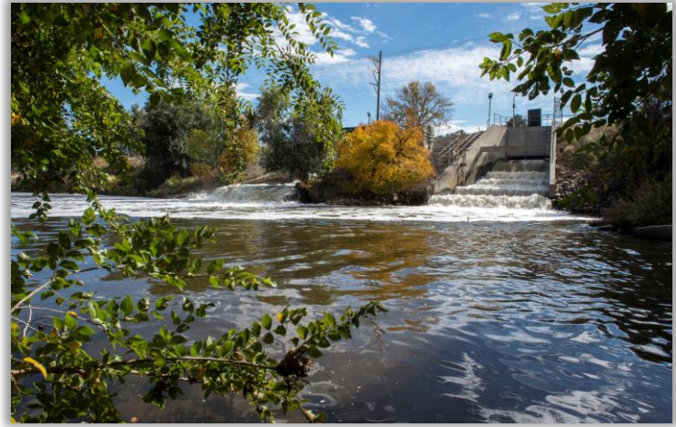
Outfall area at RWHTF, where treated wastewater (effluent) is returned to the South Platte River
