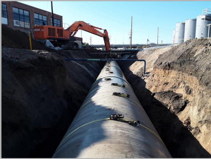
New Delgany Interceptor segment being placed beneath the NWC
