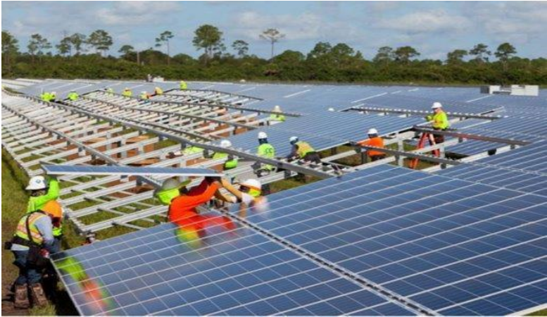
Figure 2 – Solar panel install at a wastewater facility
