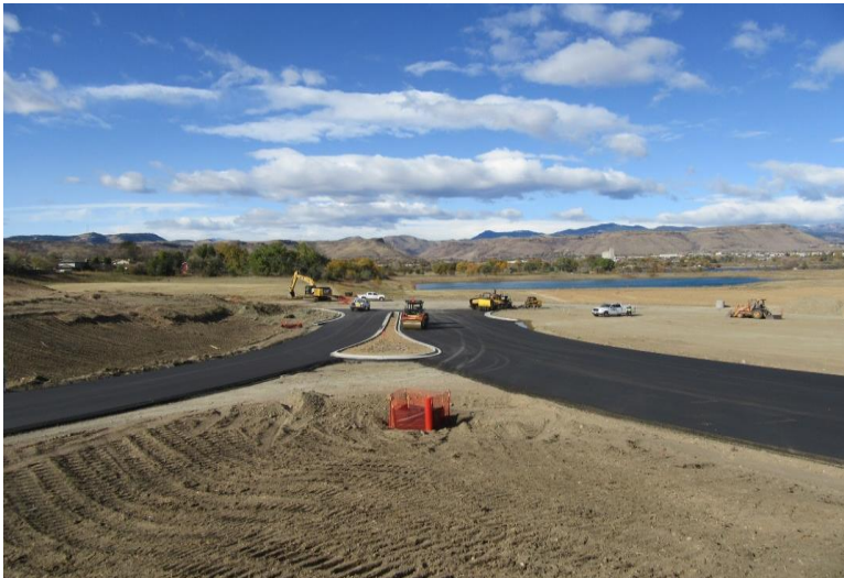
Figure 4 - New Drop Manhole between Newly Paved CDOT Hook Ramps
