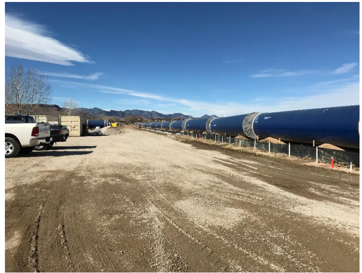
Figure 5 - 84-inch Denver Water Conduit No. 16
