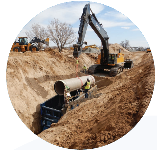
New Second Creek pipe segment being installed underground.
