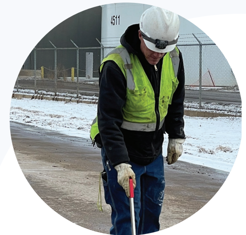
Mark Schantz, Collections System Operator, performing a utility locate.
