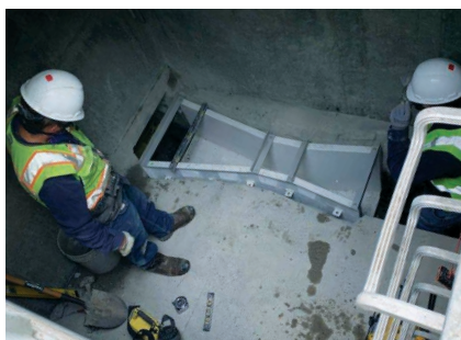
David Tatham and Chris Rowe installing the Fruitdale-Miller flume
