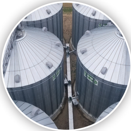
Top of new steel grain bins.
