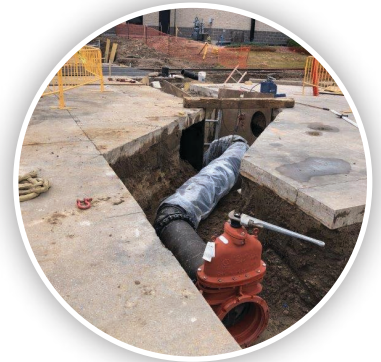
PWC line trench west of Main Street.
