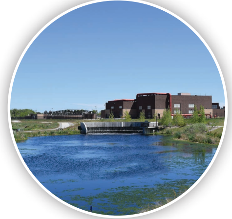
Outfalls at the Northern Treatment Plant.
