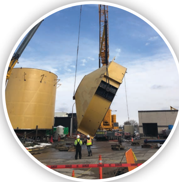
Airprex® reactor under construction at the Robert W. Hite Treatment Facility.
