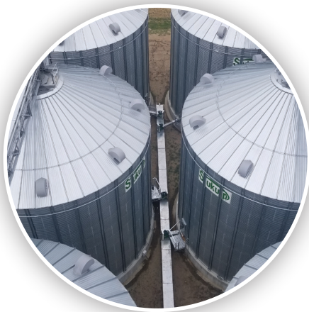
Top of new steel grain bins.
