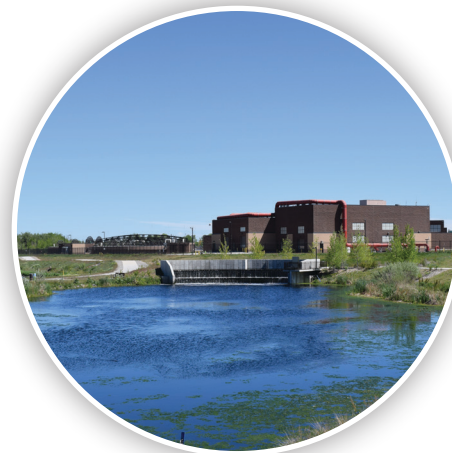
Outfalls at the Northern Treatment Plant.
