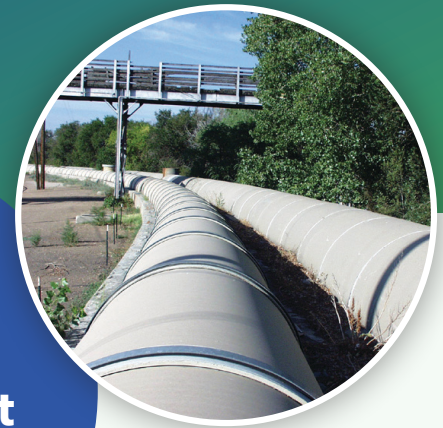
The Delgany Interceptor system replacement will be constructed underground, to allow public access to the South Platte River.
