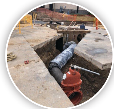
PWC line trench west of Main Street.
