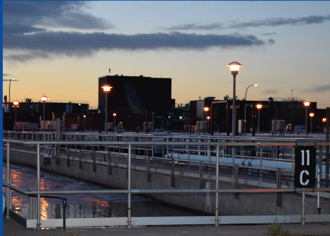
Aeration basins at the RWHTF
