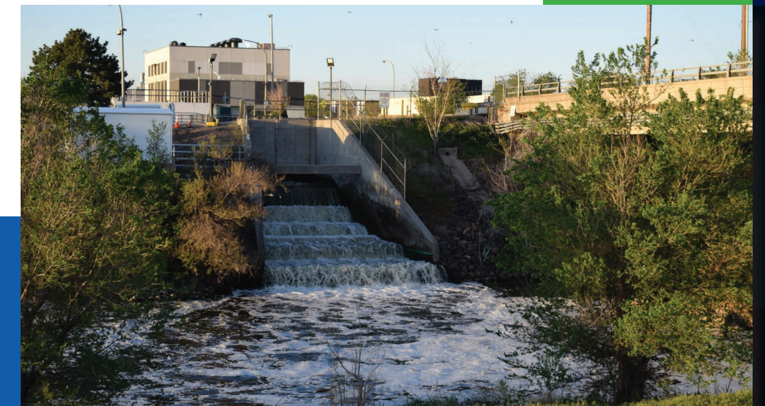
Outfall at the RWHTF
