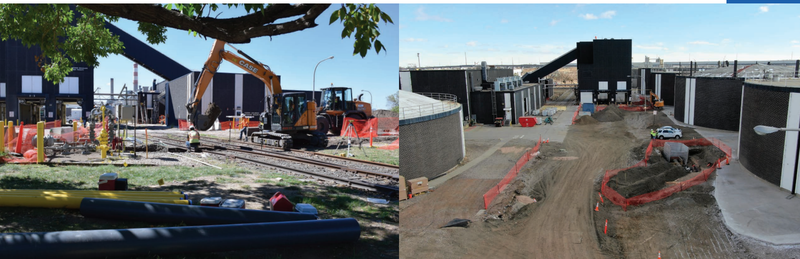
Construction for the Solids Processing Building Improvements Project
