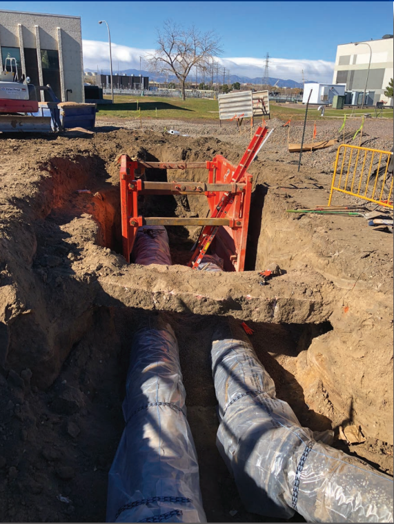
Construction for the Plant Water Chlorinated System Improvements Project
