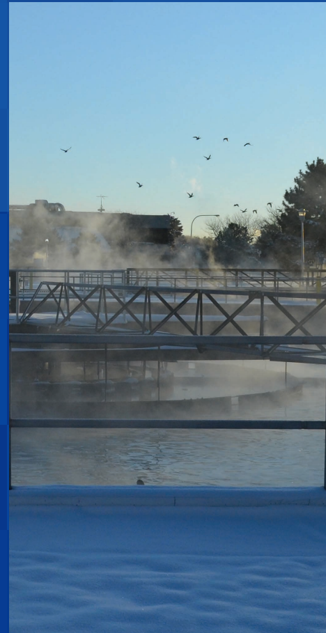
Above: Clarifier at the RWHTF Front cover (middle): Tertiary complex at the NTP Front cover (top): Grain bins at the METROGRO Farm
